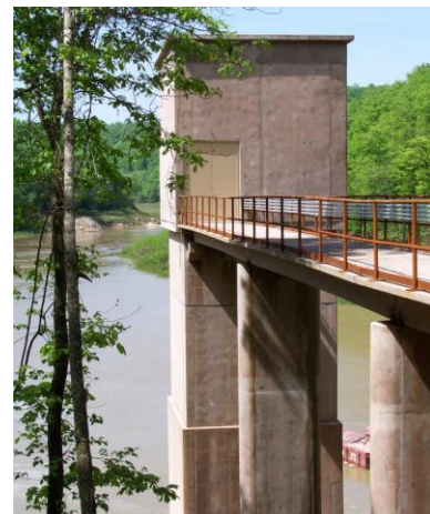
New Raw Water Intake
