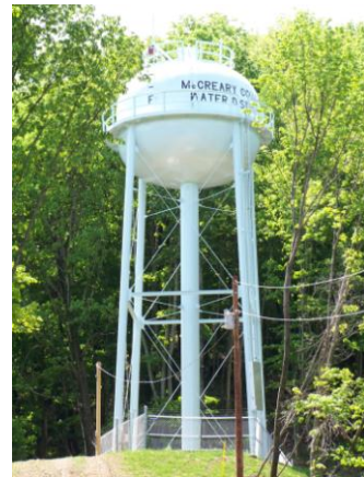
East Hwy. 92 Water Storage Tank
